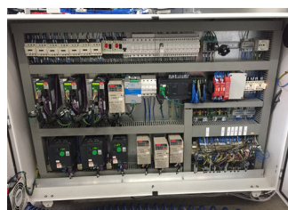
PLC with 120 In/Out, 8 servo-drives and 2 safety modules
